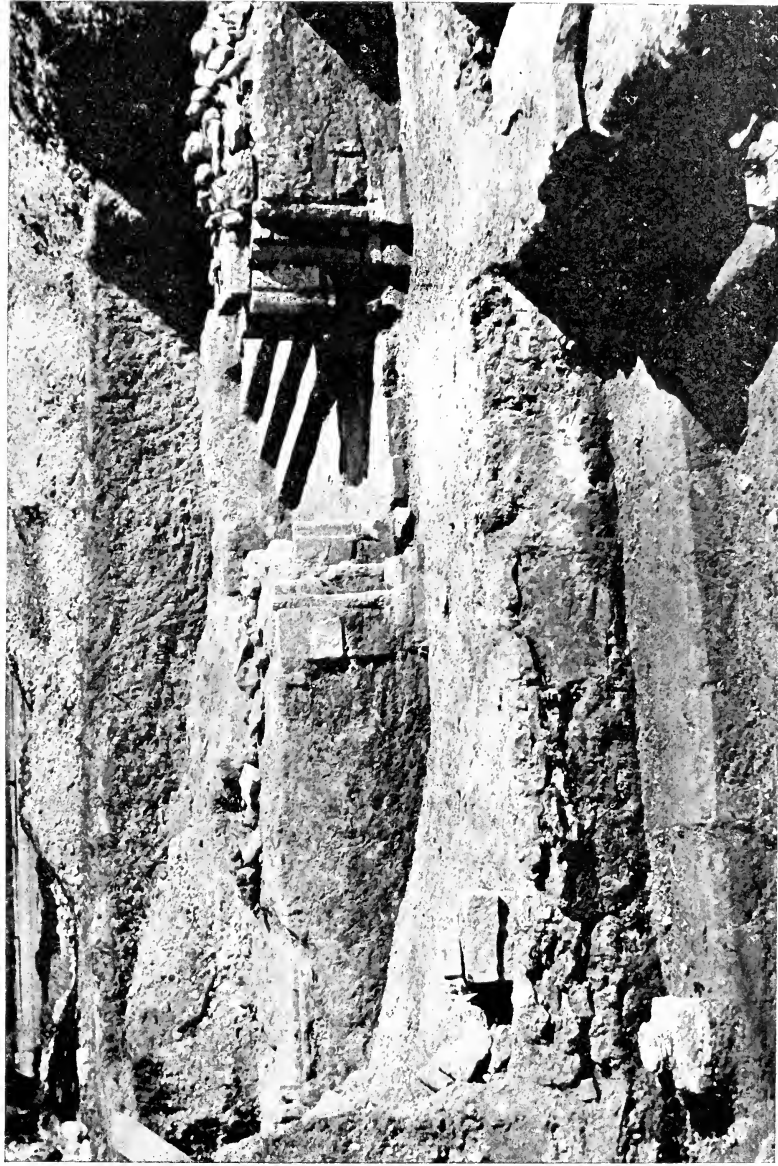
DORTER DOOR AND STEPS, WITH WALL OF CLOISTER IN FOREGROUND.
