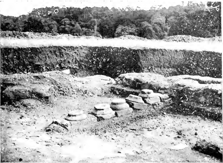
FOUNDATION WALL MADE OF BASES.
