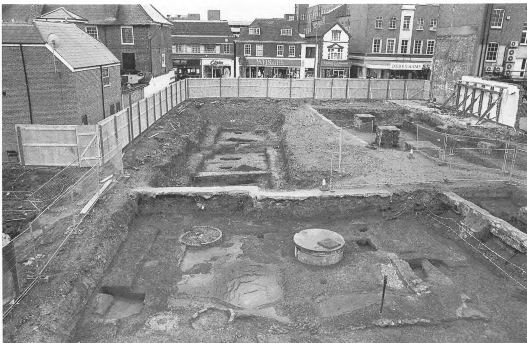
Fig 5.3 Tilly’s Lane, Staines: in the foreground, walls and red tessellated floor of a later 2nd century building; the floors soon subsided into depressions caused by earlier features. The High Street can be seen in the background. Photograph copyright Wessex Archaeology
