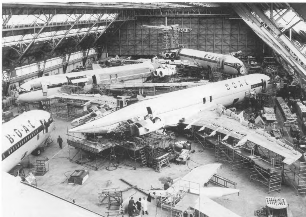
Fig 16.8 Aircraft manufacture at Weybridge showing the assembly of VC10s for BOAC and British United Airways in April 1964. Courtesy of Brooklands Museum
