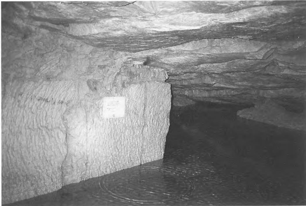
Fig 16.2 Quarry Field building stone quarry, Merstham, showing part of the Chaldon-Merstham complex of drift mines in the Upper Greensand of east Surrey. The tunnels appear to be medieval in origin but were reopened by 1807 and extended below the water table by the civil engineering partnership of Joliffe and Banks. The drainage adit no longer functions, hence the flood water as photographed in January 2001. The floor-ceiling height is generally c 1.5m. These early 19th century workings show characteristic pillar-and-stall features, with stalls or tunnels at right angles to the joint system. The pillar wall shows pick marks indicating up-dip working and distinct beds of stone, some more suitable for building than others. Spoil was backfilled underground. The notice was placed by the Wealden Cave and Mine Society to provide information on safety procedures and cave rescue during a detailed survey of the workings, of which some 17km were recorded. Photograph by Paul Sowen
